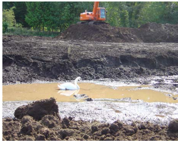
Figure 4 Stage 2: Pond excavation
