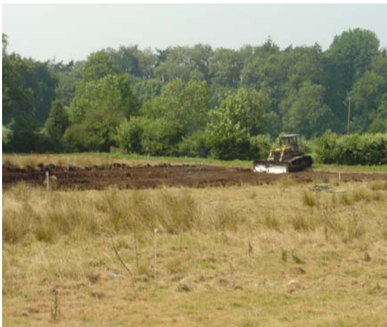
Figure 3 Stage 1: Topsoil was stripped
