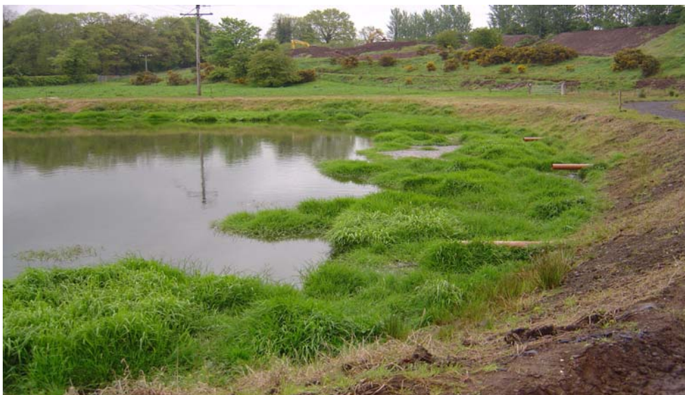
Figure 30 Grasses growing on the surface “cake” layer adjacent to pond 1 inlet pipes
